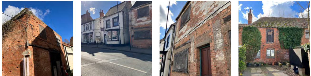
Figure 19: Derelict and empty buildings in Tuxford.
