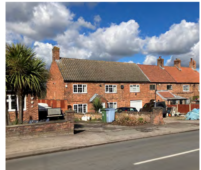
Figure 38: Masonry walls boundary treatments at Ollerton Road.
