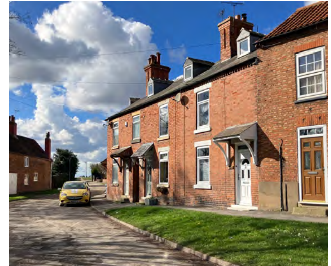
Figure 39: Open boundaries with no setback from the road at Newcastle Street / Long Lane.
