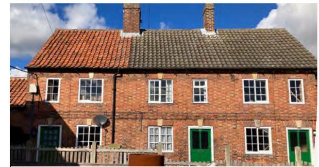
Figure 14: Flemish bond, brick banding and keystones are common on older buildings
