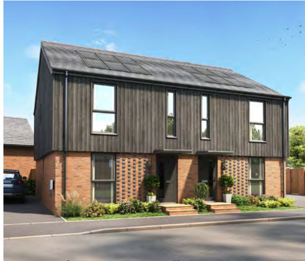
Figure 106: Carbon negative affordable homes in Derbyshire.
